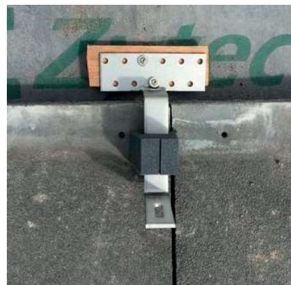
Step 2: Put SolarFlash (small) on the bracket.
