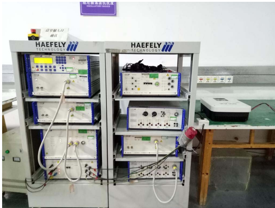
16.7.Photo of Surge Test
